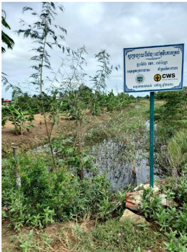
Restored Canal in Kouk Trab Village to prevent floods during the rainy season.
