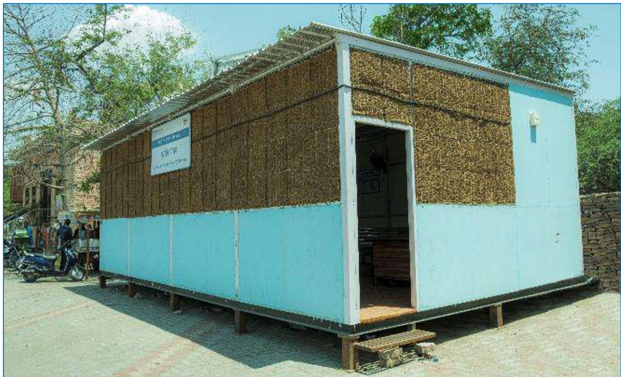
Net- Zero Cooling Station.
