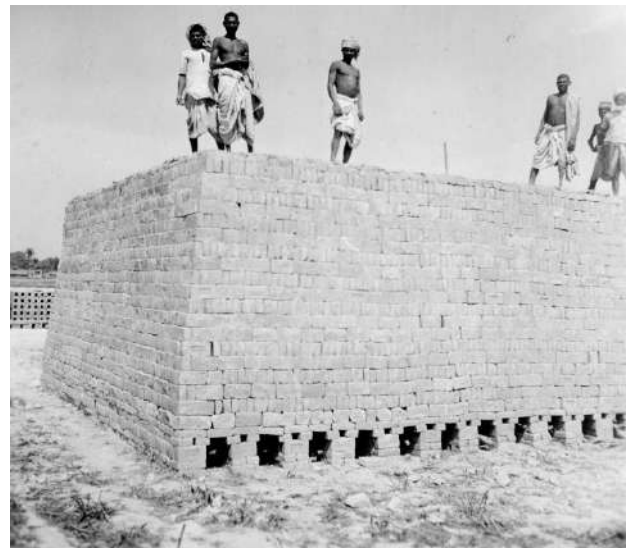
Brick kiln set up in the aftermath of the 1934 Bihar-Nepal Earthquake. Source: "SCIIA – Service Civil International – International Archives, Bibliothèque de la ville, La Chaux-de-Fonds (Switzerland)".
