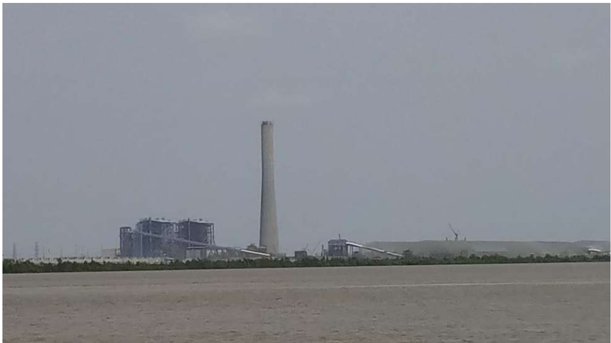
View from a coastal town showing an imposing installation for power generation.
