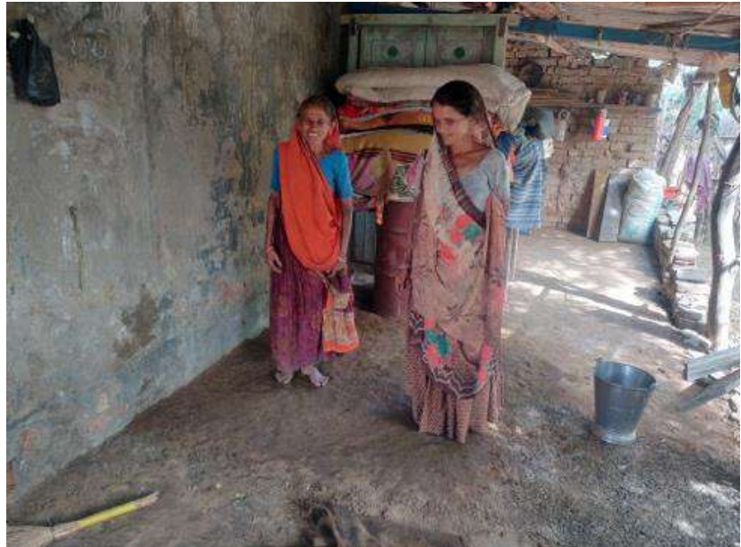
Women preparing the floor with river sand before the arrival of monsoons ( pagthi khundine lipan ) by trampling the surface barefoot, which helps to restrict insects emerging from the floor during the monsoon. Photo credit: Megha Sheth (May 2022)
