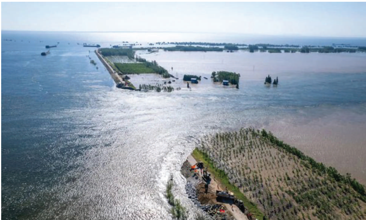
Dike flooded. During the flood in Hunan in 2024, floodwaters flow over a dike (photo from Global Times . 2024. Update: Closure Work Starts at Breached Dike of Dongting Lake in Central China. 6 July).
