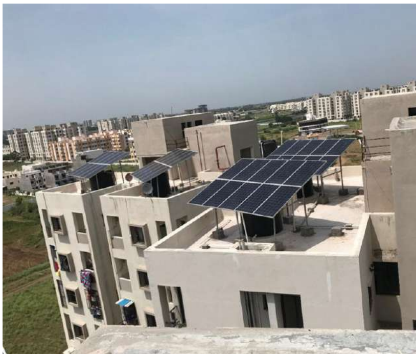
Solar PV installed as a cool roofing solution for affordable housing in Rajkot. (credit: ICLEI South Asia)
