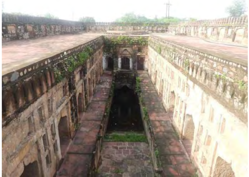
Figure 1. Chandeva ki Bawadi in Datia, built by Raja Veer Singh Judev I, is one of many traditional stepwells in the region designed to combat water scarcity and summer heat.
