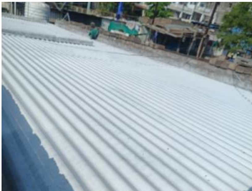
Application of Cool roof solution, Jalgaon, Maharashtra, India.
