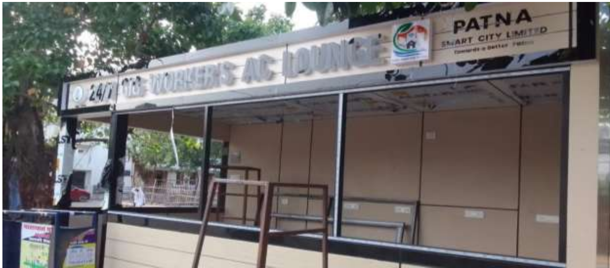
AC cooling/rest centre for gig workers during extreme heat.
